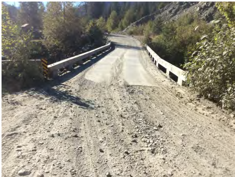
Approach from Right Bank when facing downstream
