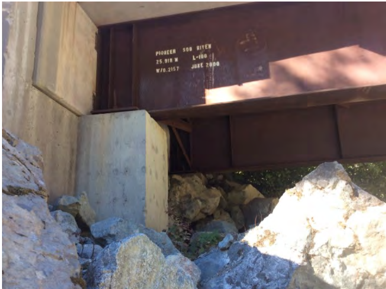
Left Bank Abutment when facing downstream
