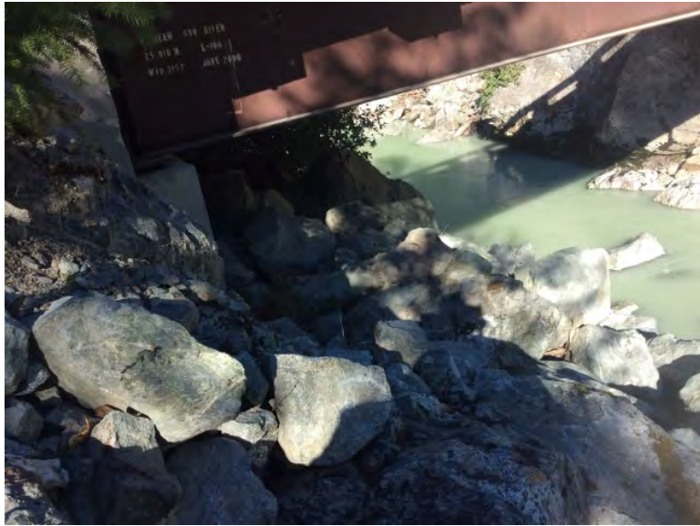
Left Bank Abutment when facing downstream
