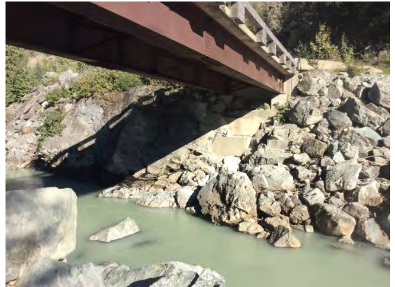
Right Bank Abutment when facing downstream
